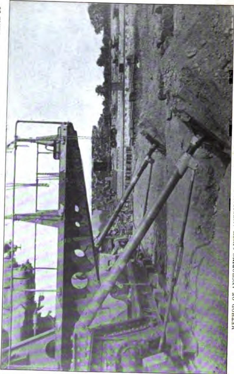
METHOD OF ANCHORING 8-INCH AMERICAN RAILWAY MOUNT FOR FIRING ACROSS TRACK.
