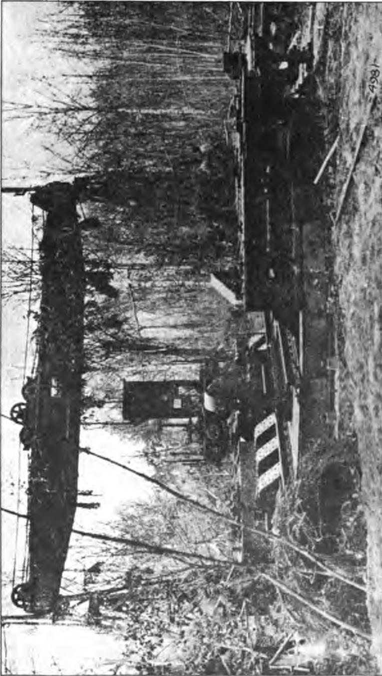
GANTRY CRANE USED IN INSTALLING EMPACEMENT FOR 380-MM. GERMAN GUN MOUNT.
