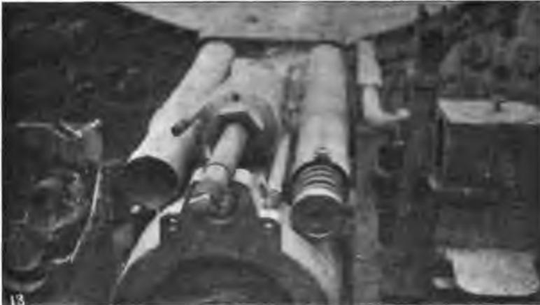
CRADLE RECOIL CYLINDERS AND RECUPERATORS OF THE 17 CM. BATTERY
