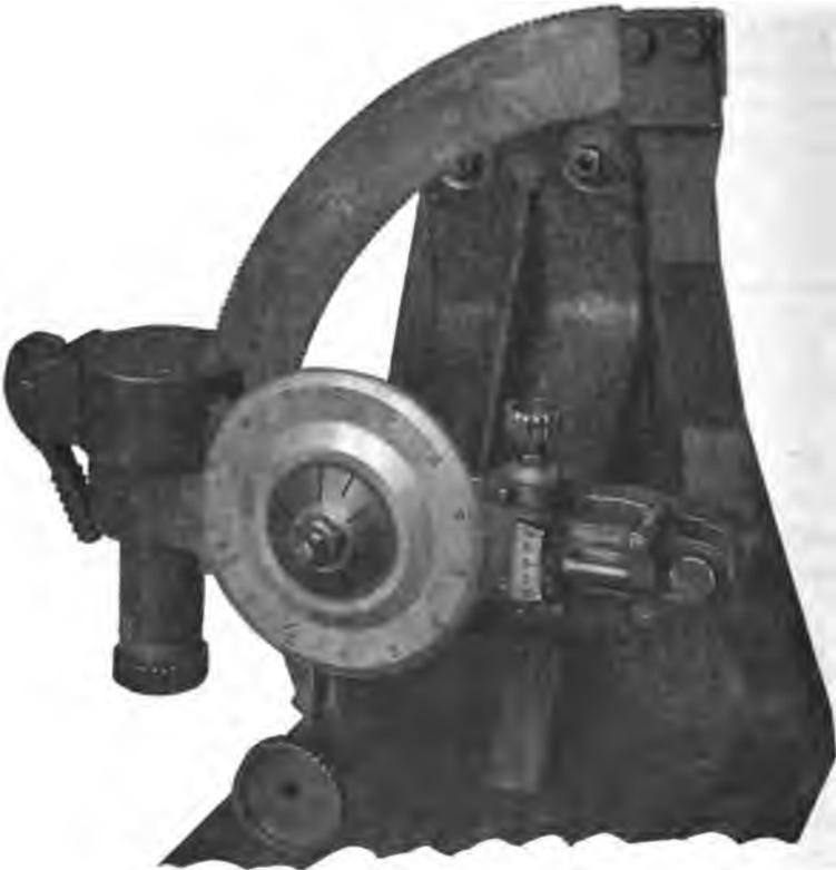
STANDARD ELEVATION QUADRANT USED WITH ALL RAILWAY MOUNTS.
